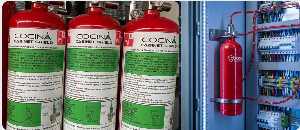
"A compact, standalone fire suppression system designed to protect electrical cabinets, server racks, and enclosed machinery."
